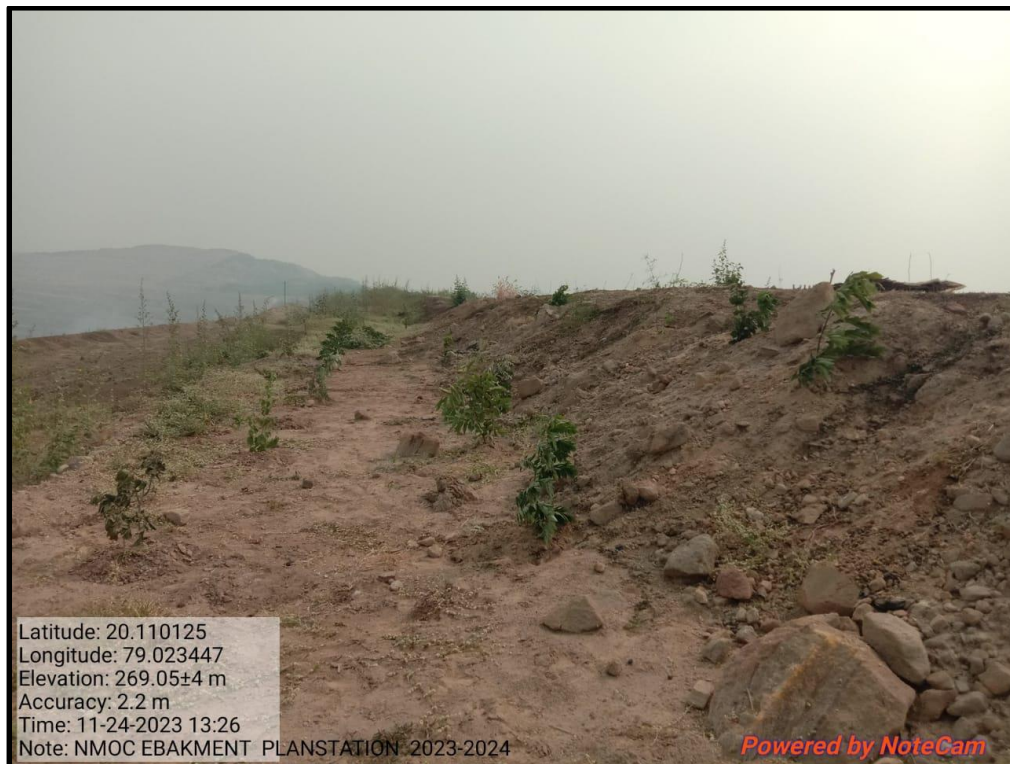
Photograph-8: Plantation on Embankment (New Majri OCP)
