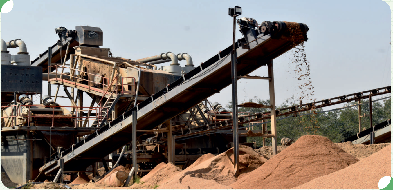
■ Sand Segregation Plant in operation.
