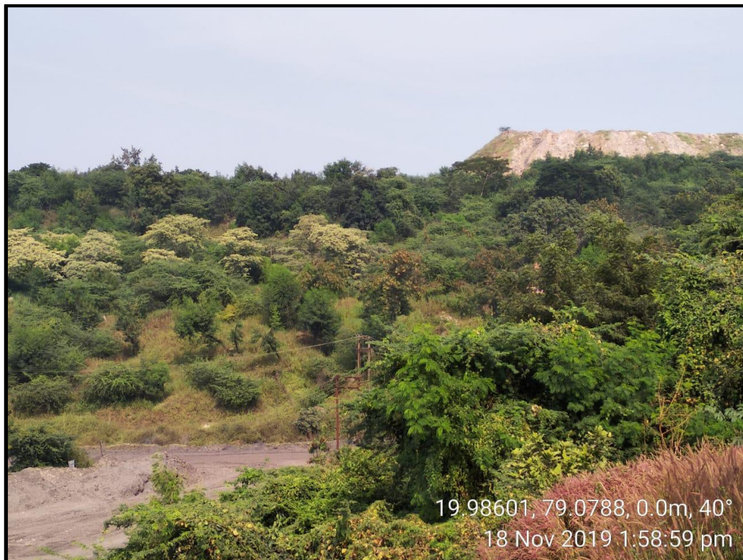
Photograph-7: Plantation OB Dump (Niljai OCP)
