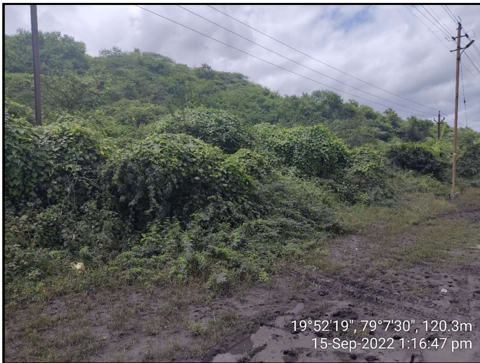
Photograph-4: Plantation on Embankment (Mugoli OCP)
